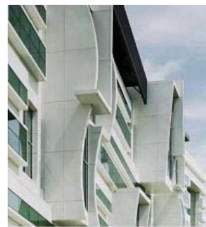
"Pods" enliven the aluminum-and-glass façade of the RPCI building. These projecting spaces house informal lounges where scientists can gather.
